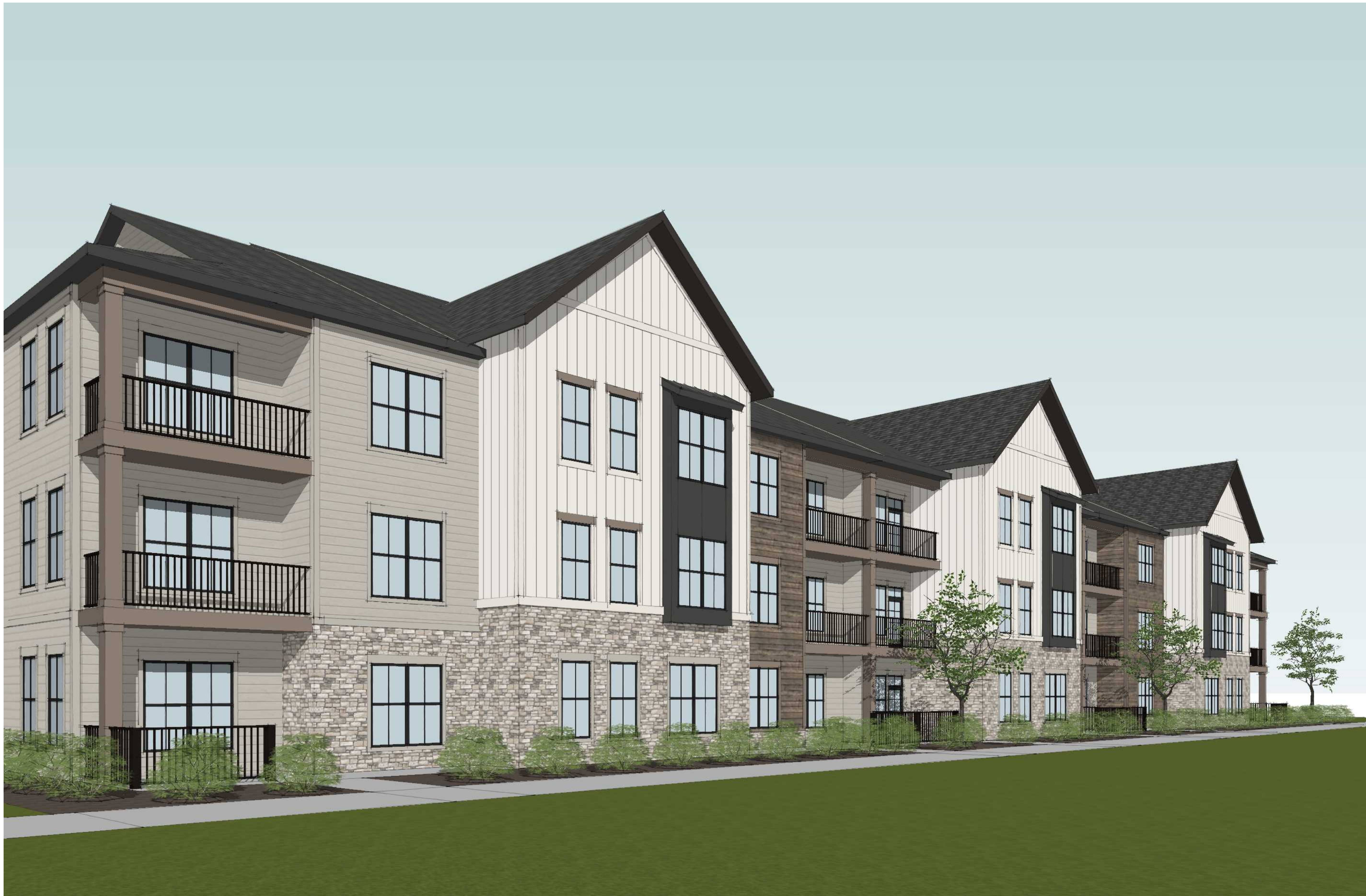
VIEW LOOKING AT APARTMENT BUILDING TYPE B 3-STORY REAR ELEVATION
