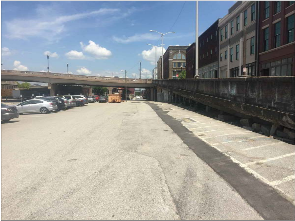
Primary Entrance from City of Knoxville Parking Lot
