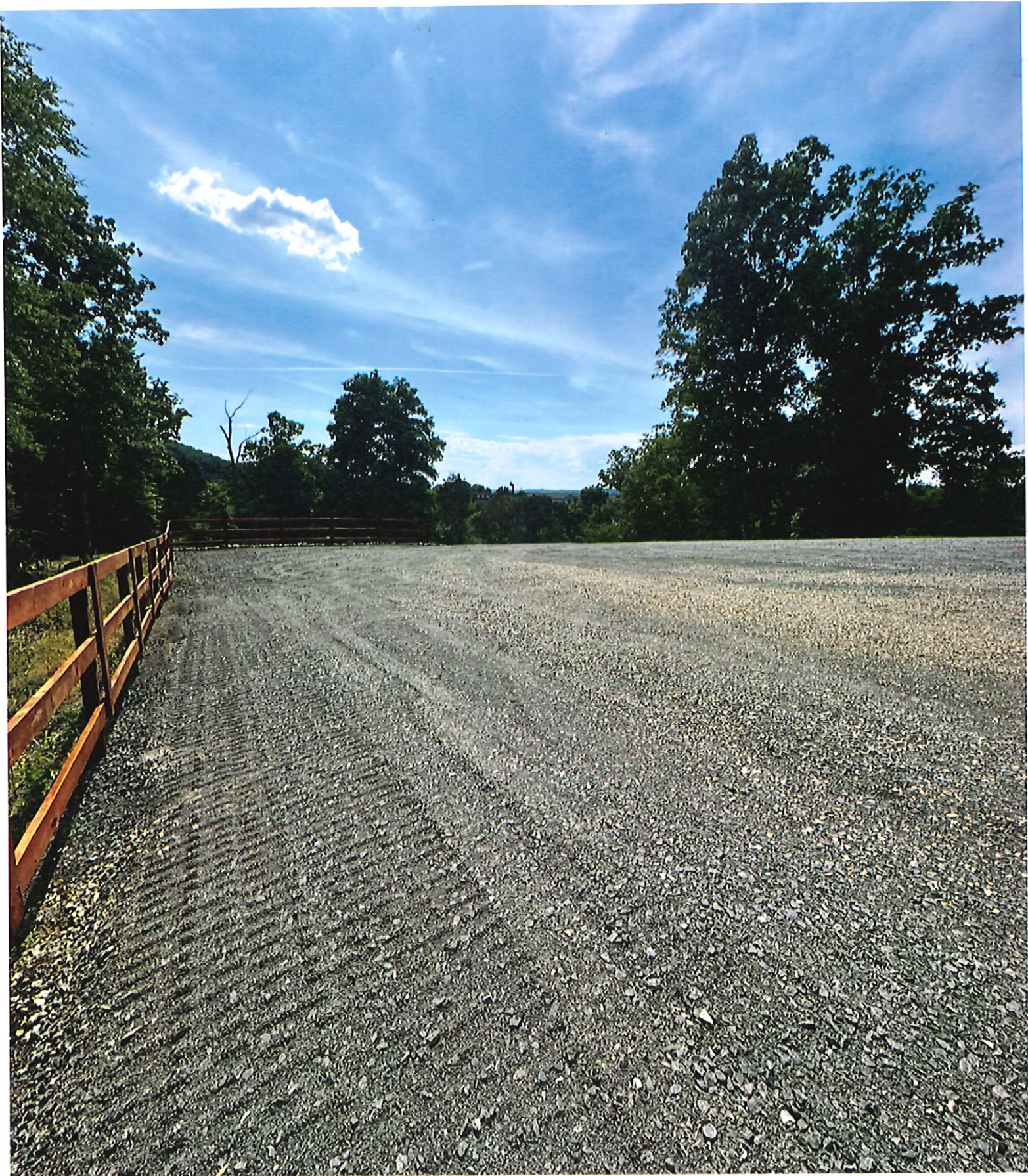
Upper Parking lot
